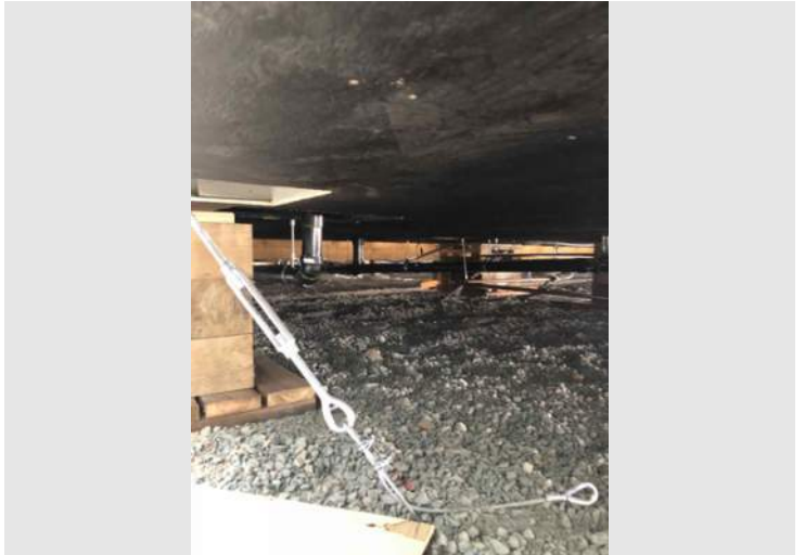
Description Plumbing and gas rough-in below building
