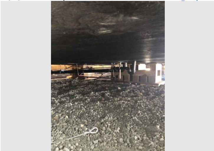
Description Plumbing and gas rough-in below building
